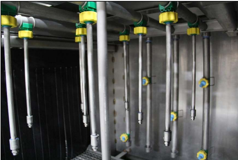
Wash zone with extended spray nozzles
